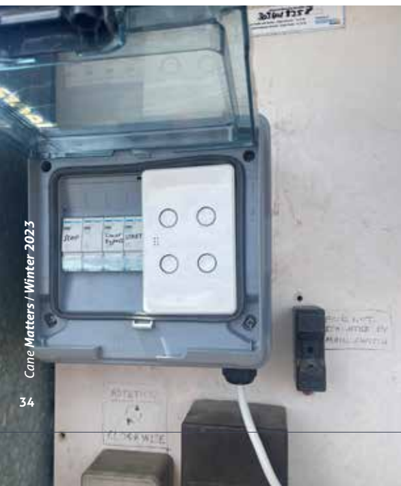
Wifi pump controller using a four-button smart light switch.
