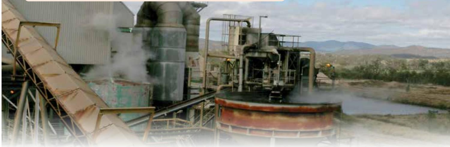
The power station will use bagasse to produce 24 megawatts of electricity – enough to power every house in the Tableland region.
